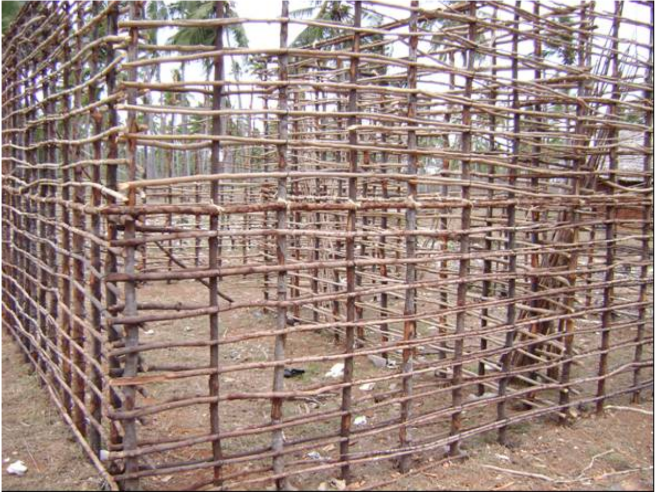
Plate 2. Traditional house, composed virtually of mangrove poles, under construction (Photo; J. Lang'at)
