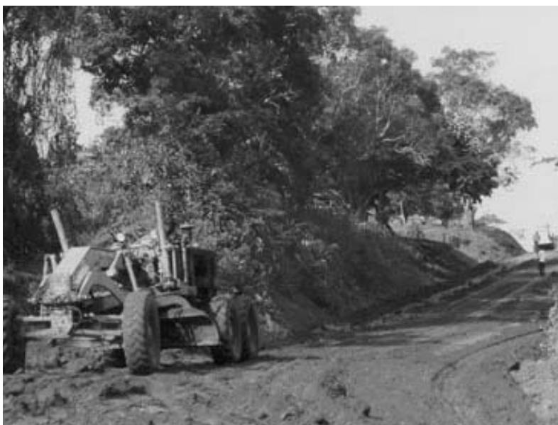
Along Mbang - Lomie road reconstruction. In Cameroon also, road are suffering.
