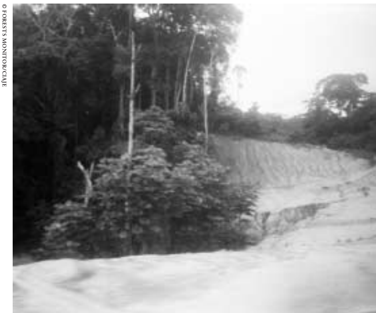
Erosion caused by logging
