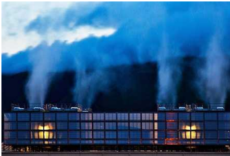
Google data centre. Ph: Green Queen
