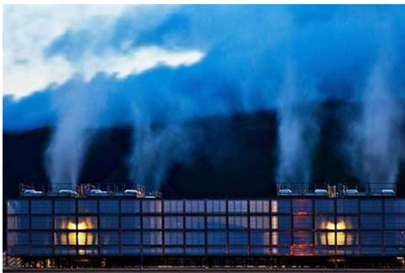
Google data centre. Ph: Green Queen
